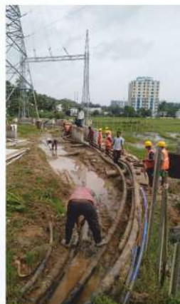
EHV 220 kv UG-XPLE Cable Laying for KSEB at Kaloor Sub-Station - Kochi
