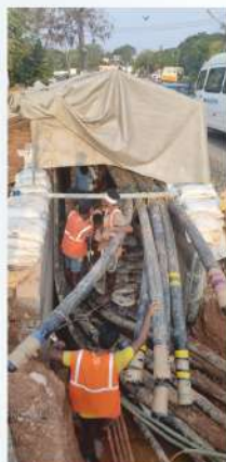
EHV 220 kv UG-XPLE Cable Laying for KSEB at Kaloor Sub-Station - Kochi
