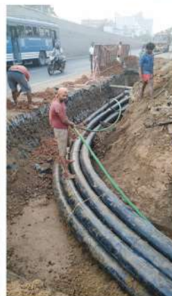
EHV 220 kv UG-XPLE Cable Laying for KSEB at Kaloor Sub-Station - Kochi
