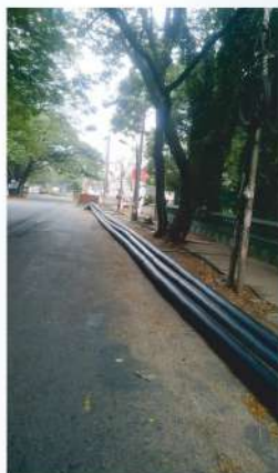
EHV 220 kv UG-XPLE Cable Laying for KSEB at Kaloor Sub-Station - Kochi
